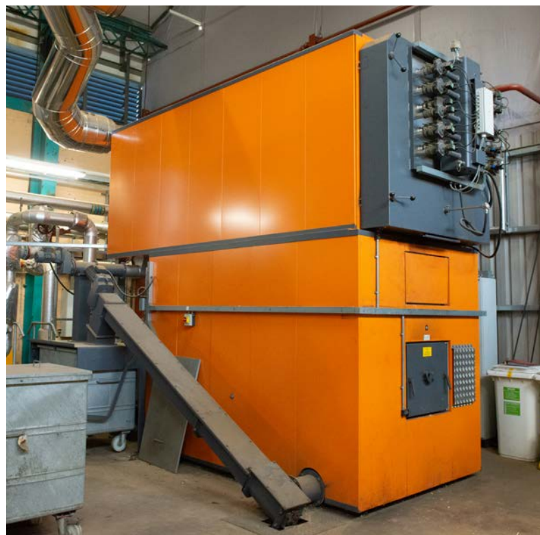
Biomass boiler in our Energy Centre, governed by OFGEM under the Renewable Heat Initiative (RHI)
