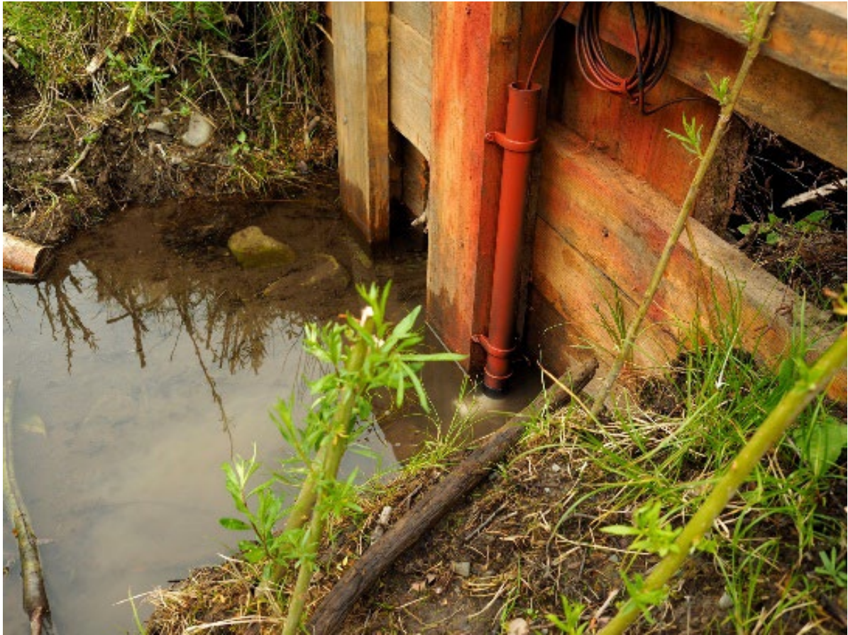
Figure S2. One of the adjustable wooden sluices through the Enhanced Hillslope Storage (EHS) features at the Birds Park NbS trial site, near Kendal town, Cumbria (UK).
