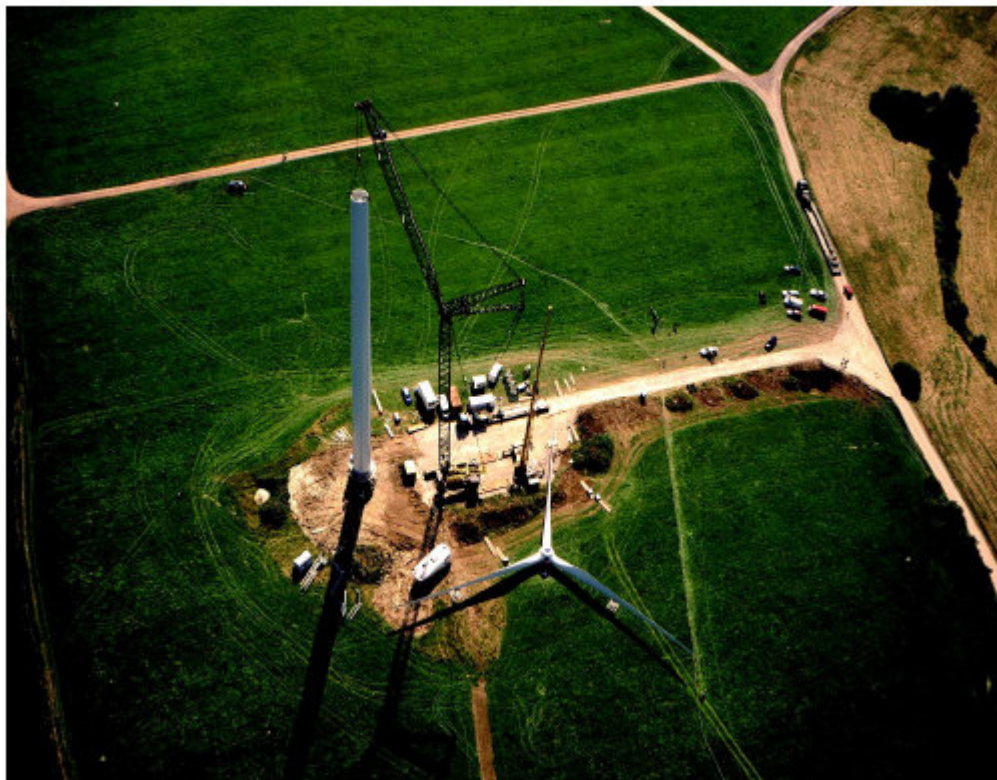
Photograph 2.1: Construction Areas at Turbine Installation
